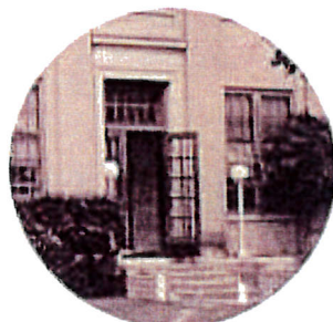
Original wood doors (left) and wood sash windows (right)
