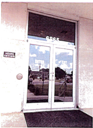
Aluminum and glass doors at north entry
