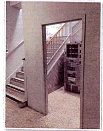
This partition wall was added to the south staircase to create a small break area with vending machines
