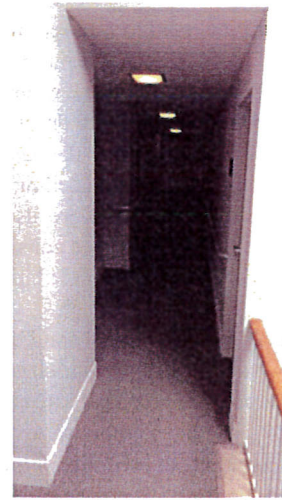
Second floor stairwell ceiling
