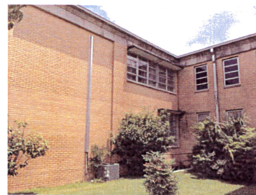
The walls of the east wing
