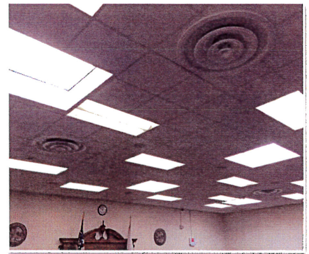
Second floor, historic courtroom ceiling and skylights
