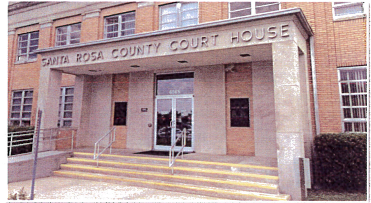
The concrete porch, or portico, on the north facade of the courthouse
