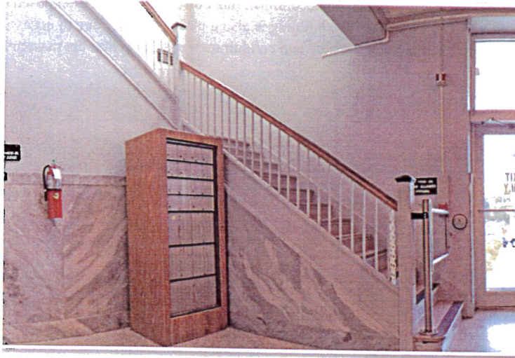
This original staircase by the north entrance features a newel post and balustrade made of cast iron and marble stair treads
