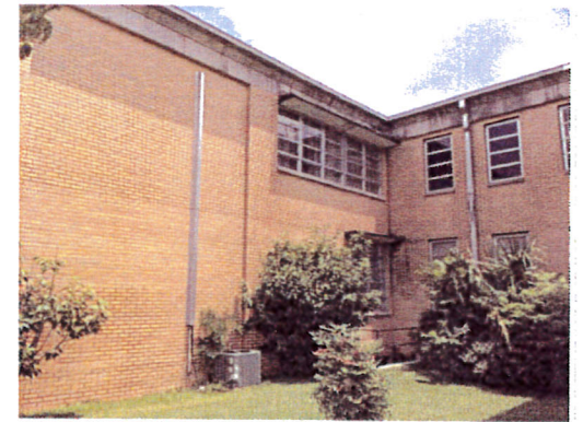
The walls of the east wing
