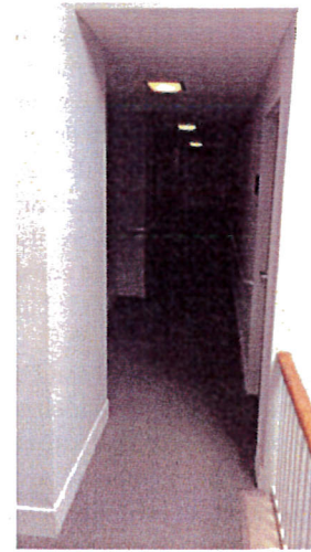
Second floor stairwell ceiling
