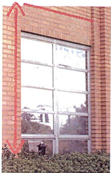
Aluminum windows on the first floor. The red lines indicate the original window dimensions. Note the brick infill.
