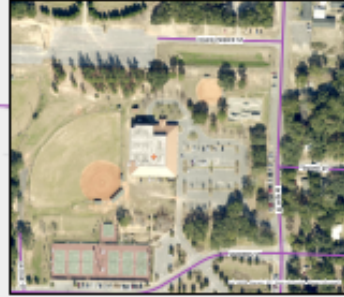
Community Center Existing Site Conditions
