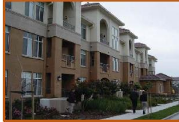
Landscape strip between road and sidewalk enhances pedestrian environment
