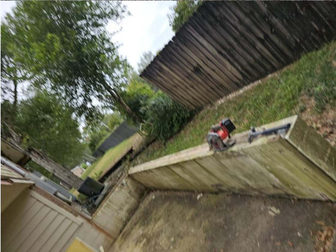
Previous fence pictures.
