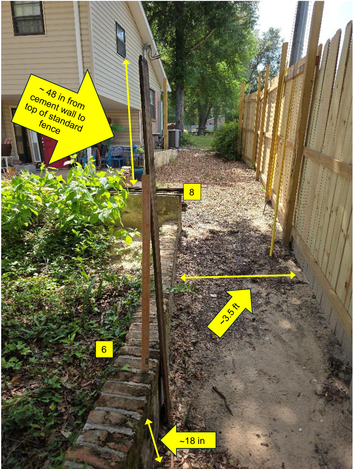
Area (6) showing brick wall height of 18" with 36" yardstick on top and standard 6ft fence panel height. This is 3.5 feet from new fence location.
