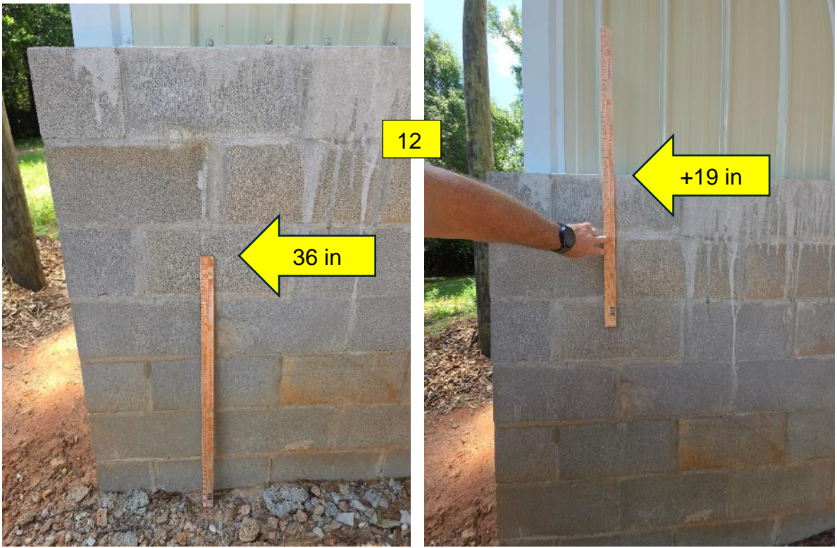
Area (12), lower rear corner is 55" tall
