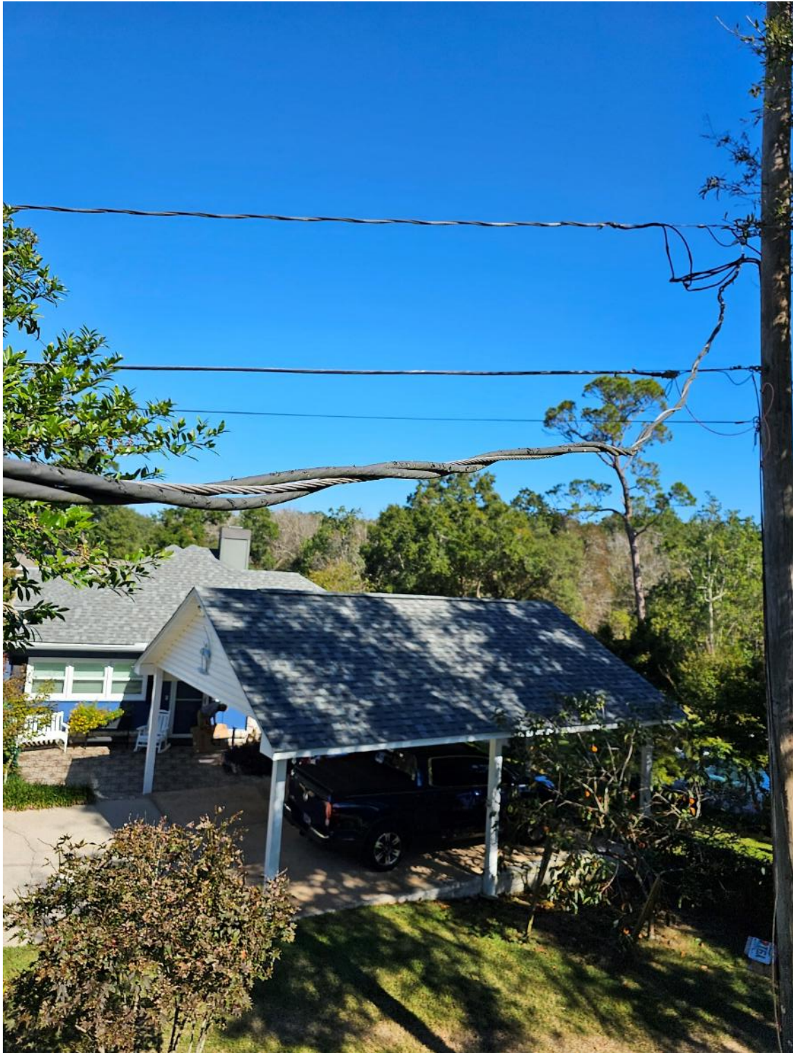
Reference picture showing how/why I have pictures of their camera. I was photographing the powerlines for the power company where squirrels have been chewing.
