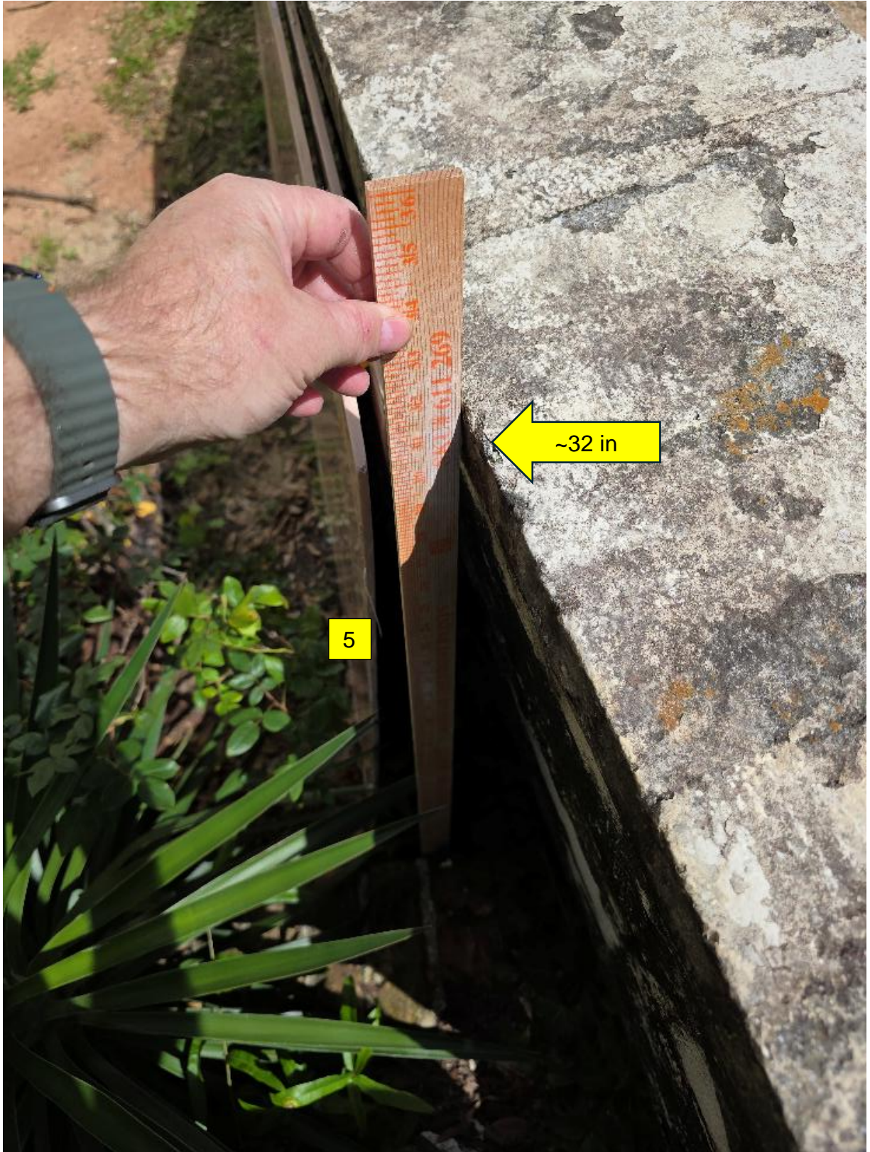
(5) Outside wall height of 32". This is outside of area labeled (4)
