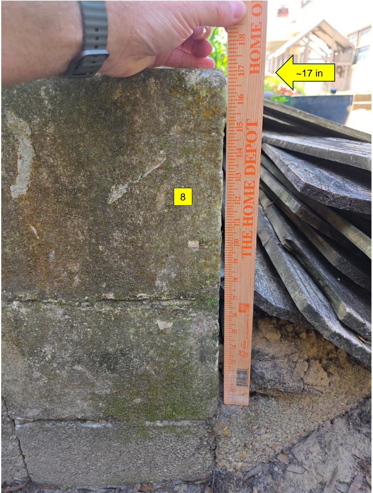
(8) view and measurement of front of wall on the edge of the patio, near where the fence will be located
