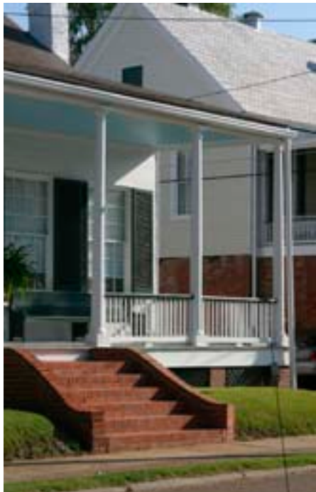
Concrete sidewalk and brick steps
