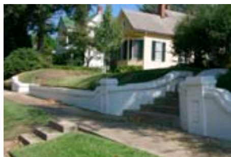
Low, painted masonry walls edge the sidewalk
