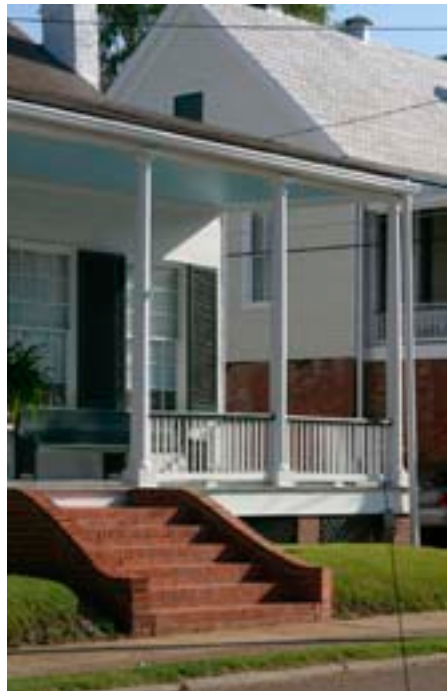
Concrete sidewalk and brick steps
