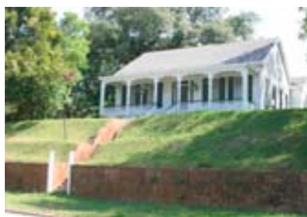
Brick wall and steps
