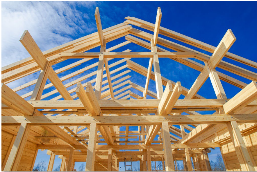
New Housing Construction
