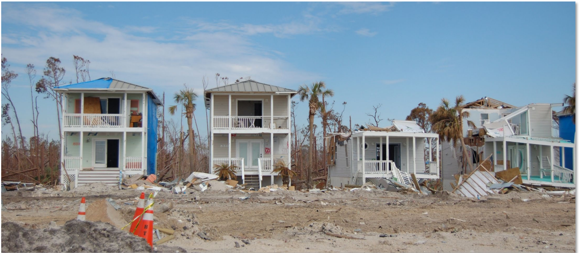
Hurricane Michael damage in Mexico Beach
