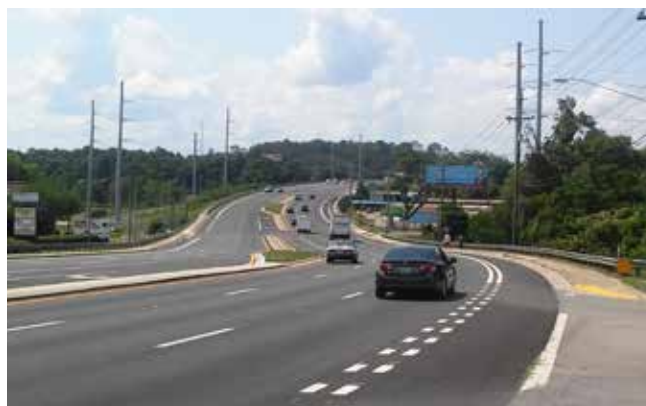
Narrower travel lanes help manage speed and provide for wider bike lanes. Location: Capital Circle NE, Tallahassee, FL Source: FDOT
